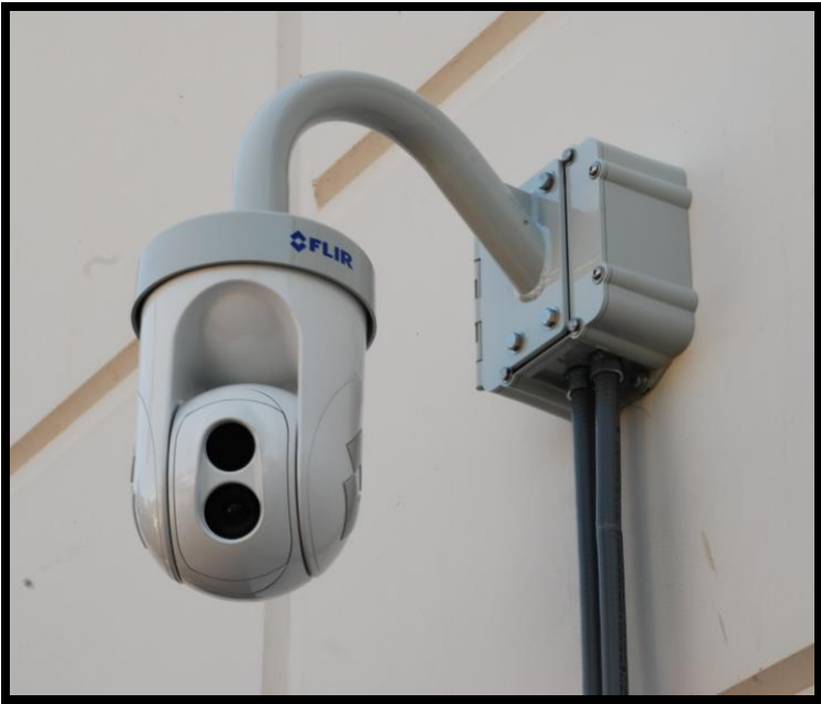
Shown with dual conduits on building surface
