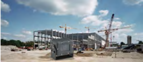
Construction machinery and cranes
